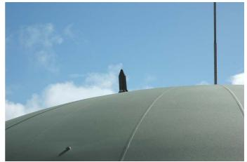
The Rain Alert<sup>™</sup> wireless tank level monitor is fitted to a tank system at the RWRC and transmits a reading of tank levels to a Receiver located in the Engineering Faculty over 150m from the tank.
